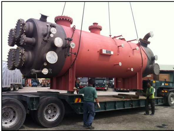
The 24 M/Ton boiler being loaded on 2-axle low-bed trailer.
