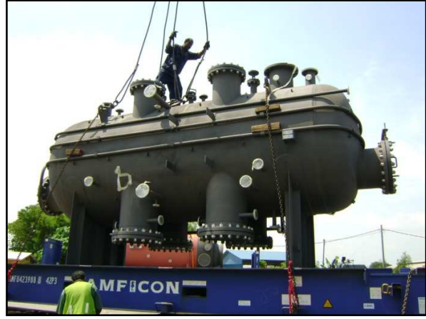
Un-stuffing of the SRU boiler unit from flat-rack container.
