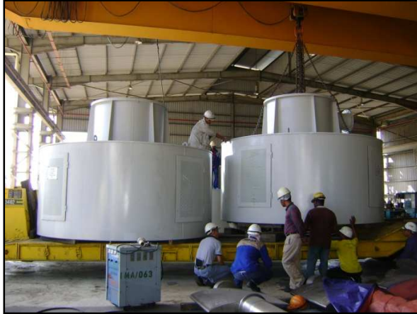
Machine Top units being loaded on 2-axle low-bed.
