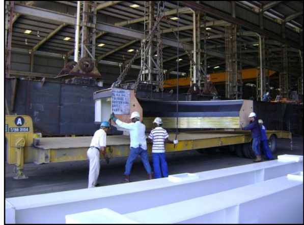
The 28.00 M/Ton Bottom Ring carefully loaded on 2-axle low-bed.
